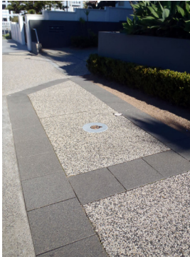
Nodal section pathway with an exposed aggregate concrete finish.
